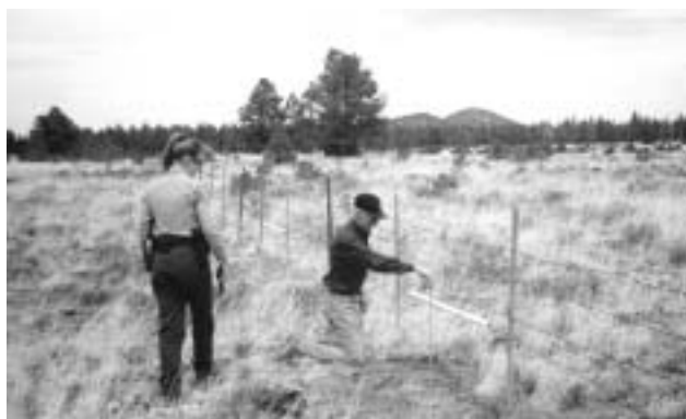
Bill Humphrey of the Arizona Department of Transportation and Velma Holt of the Arizona Game and Fish Department install goat bars to help pronghorn travel freely under fences along a stretch of Highway 180, known as an important pronghorn corridor.
