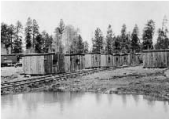
Small mobile buildings, as shown in this historic photo, were carried to logging sites by train to form a temporary village.
